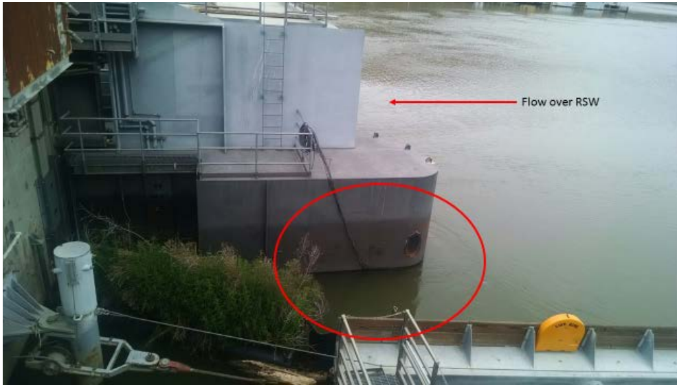
Photo 1. Southeast corner of RSW and northeast corner of forebay debris boom.
